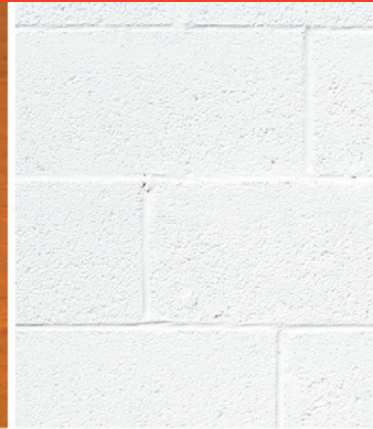
Painted Cinder Block or Concrete
