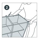
Place the base cabinets roughly in the position they will be fitted and according to your kitchen plan. Use a spirit level to mark a vertical plumb line to simulate the sides of each cabinet.
