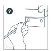
Start by fitting the corner wall cabinet. Hold the wall brackets in position and mark through the holes in the bracket
