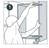
To decide the height, make sure you're clear on how you'll position the cornice pelmet and how it joins to your end panel. Clamp panel into place with 2 cm overhang at the front edge.
