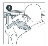
Drill through from the back with a piece of timber clamped to the front of the door. This prevents the drill bit from damaging the finish.
