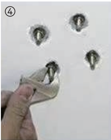
④ Tighten with a spanner.
