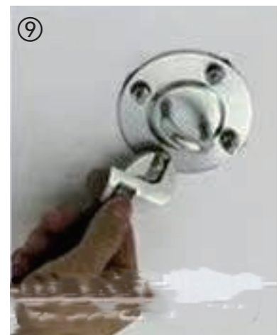
⑨ Tighten with a spanner.
