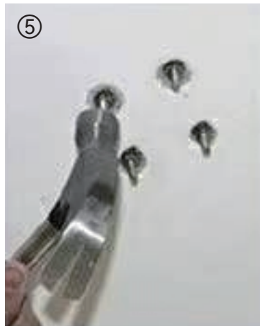
⑤ Tap the screws with a hammer.
