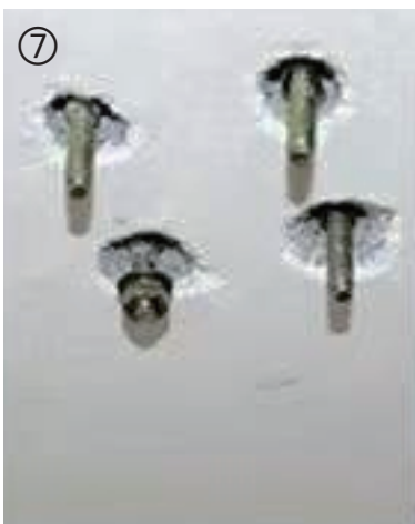
⑦ Remove the nuts and washers.
