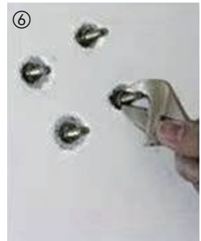
⑥ Tighten the screws with a spanner to expand them.
