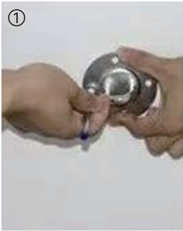
① Marking the location of drilled holes in the ceiling.
