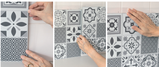
Apply the next tile, overlapping the clear membrane to form a waterproof barrier between the tiles.
