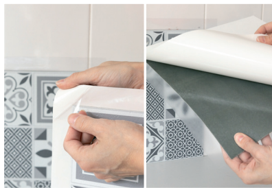
Peel away white backing paper (leaving the clear membrane in situ).
