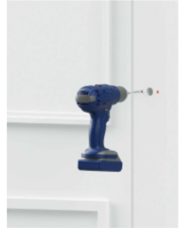
6. Drill Bolt-Through Holes
