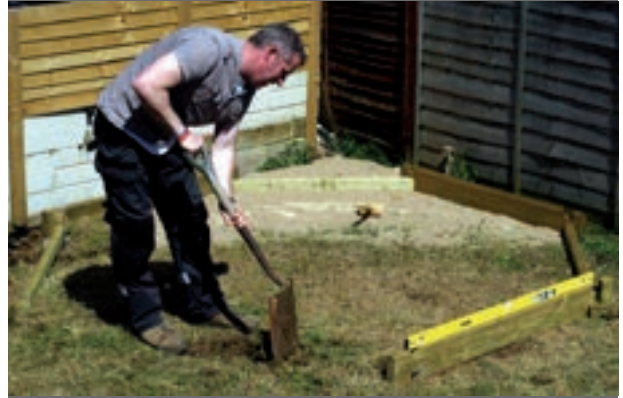
Prepare the ground
