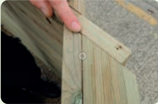
Top view of Shelving Support in place
