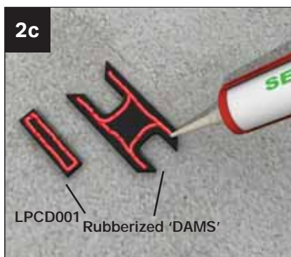
2c Take 'rubberized' sealer strips and generously butter with silicone.
