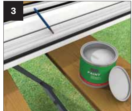
3 Finally, apply an air drying top coat with a fine brush.
