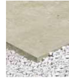
Dry laying on gravel
