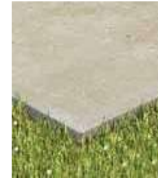
Dry laying on grass
