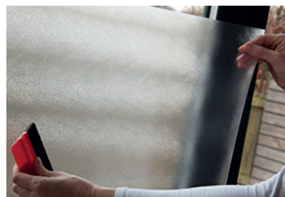
Apply onto the glass and slide the vinyl into place leaving a gap away from the edge. Use a d-c-fix smoother or squeegee to remove any excess water.
