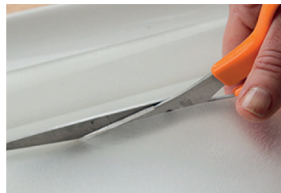
Cut the vinyl 2mm smaller than the window, this ensures the vinyl is not touching the edge or seal.
