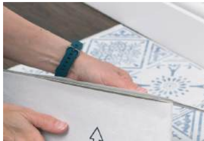
Snap the tile back to remove the cut piece
