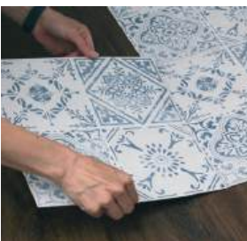
Butt join the tiles and stick to the floor
