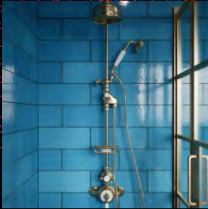
SEALING AROUND BATHS, SHOWERS, SINKS AND TOILETS.
