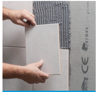
TILING WALLS & FLOORS
