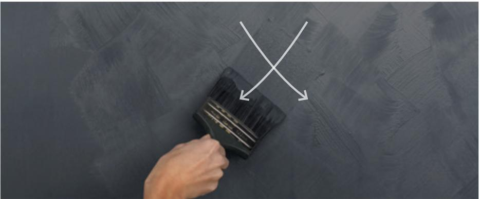
For the second coat, apply the Chalkwash with a wide, soft brush at alternating angles in a "criss-cross" manner.
