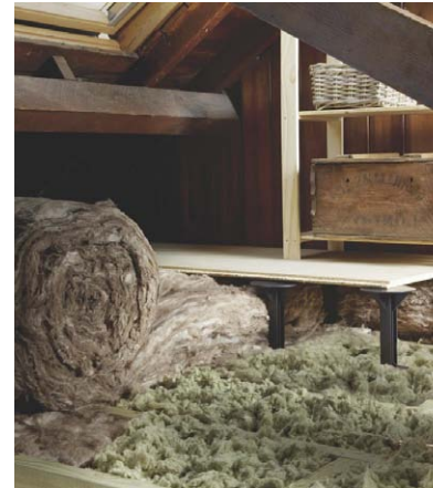
Loft stilts enable customers to fit boards over insulation so they can still use their lofts for storage
